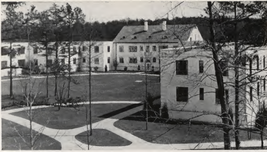
Top —Example of housing project privately financed with FHA-insured mortgage. Country Club Apartments, Greensboro, North Carolina. Concrete floors and concrete masonry walls and partitions make this group thoroughly firesafe. Exposed lightweight concrete masonry used for interior walls of halls and stairways—for good appearance, low maintenance and high sound absorption. Charles C. Hartman, architect. George W. Kane & Co., builder.
